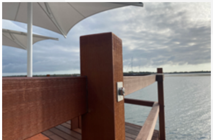
Grade 316: Stainless Steel Grade 316 is the preferred choice for use in and close by to marine environments due to its better corrosion resistance.
