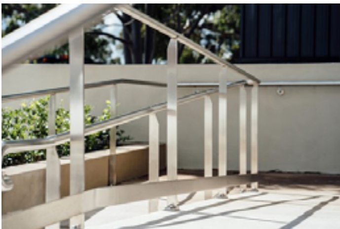
Grade 304: Stainless Steel Grade 304 resists rusting and corrosion, whilst offering durability.
